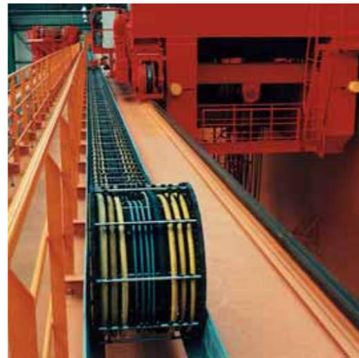
318 for long travel distance on a crane application.
